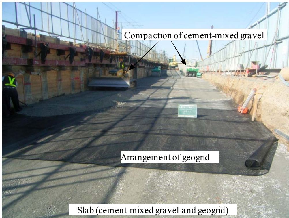
Figure 8. Application of the proposed method to the construction of railway embankment on soft ground
